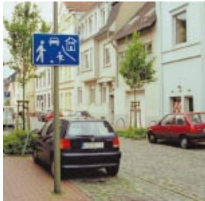
Fig. 37: Road covered with permeable surface in a residential area
