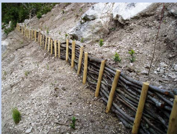
Rehabilitation of degraded slopes in the “Grands Goulets”.
